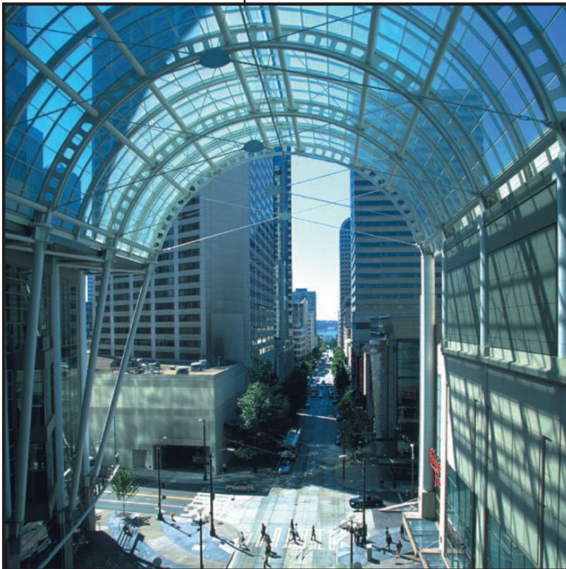
A stunning arch with usable space connects old and new exhibit areas at the Washington State Convention and Trade Center. Set in the heart of downtown Seattle, the center is within easy walking distance of more than 6,000 hotel rooms.
