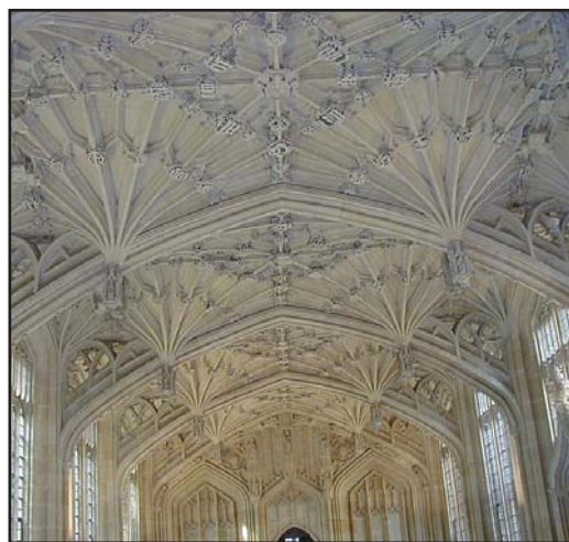
The Divinity School, which was part of the original Bodleian Library, features an elaborate fan-vaulted ceiling.
