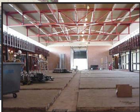
A trench for network wiring is cut into the floor of the Reading Room, which looks like an abandoned warehouse.
