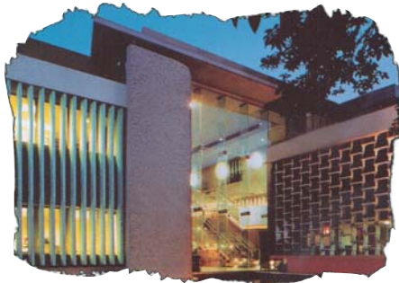
The University of Puerto Rico Law Library's exterior at night illustrates the interplay between light and shadow as well as exterior and interior decor.
