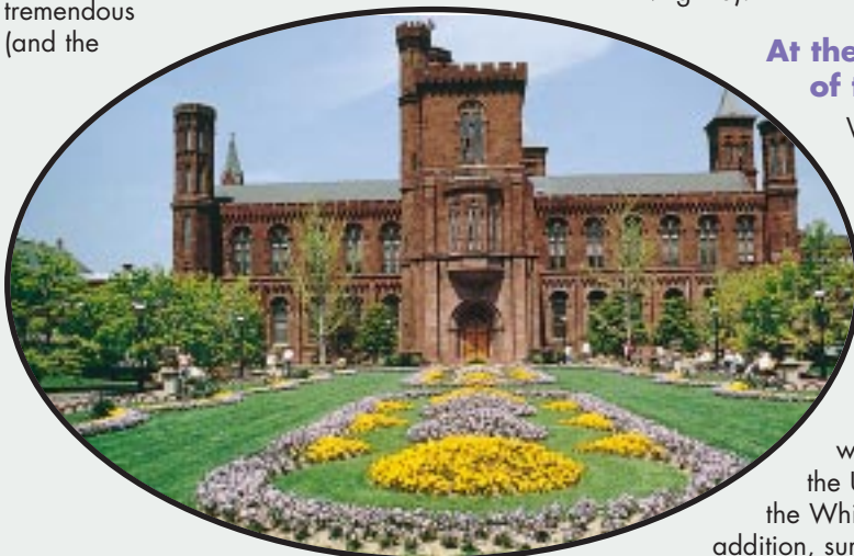
A side view of the Smithsonian Institution Building, popularly known as the Castle, which was originally completed in 1855.
