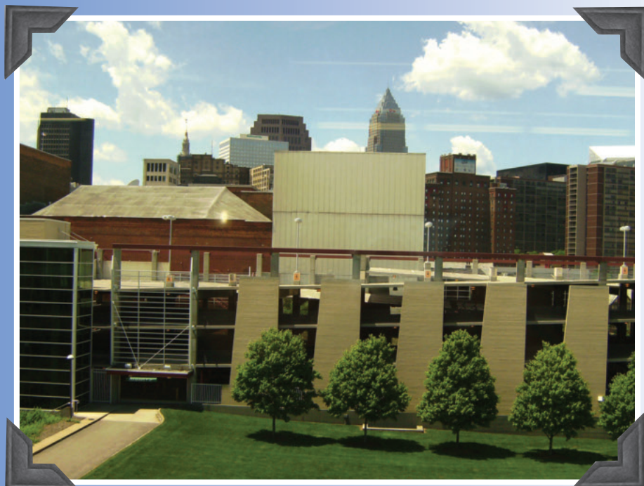
View from the second-floor study area of Cleveland-Marshall College of Law Library at Cleveland State University in Ohio. Photo by Tom Hurray, evening/weekend supervisor.
