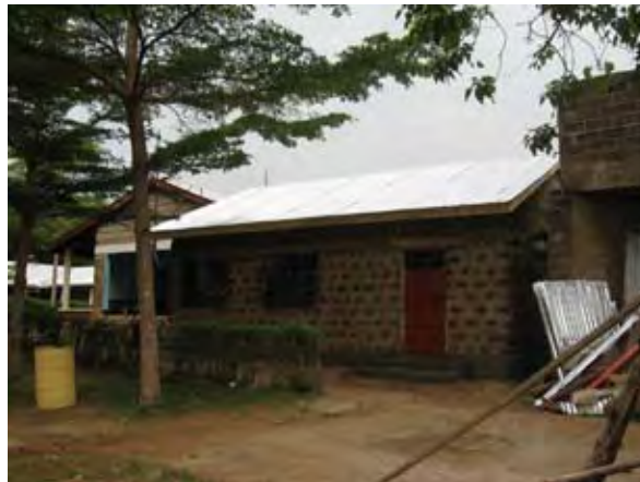
The Lwak Library Building on the grounds of the convent
